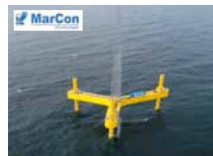
MarCon Jack-up for offshore wind power industry delivered 2012
